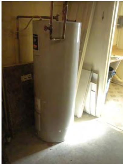
Domestic hot water tank serving the laundry area
