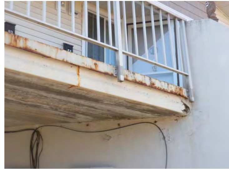
Balconies exhibit cracking deteriorating concrete and rusted railings and trim.
