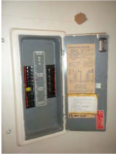
Federal Pacific Electric circuit breaker panel
